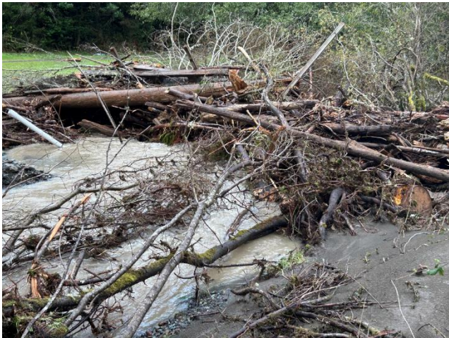
Downed trees and debris from the washed out bridge broke the water supply pipe at Indian Creek hatch house.
