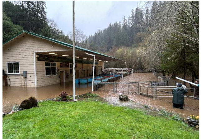
March 16 flooding at the Morgan Creek facility.
